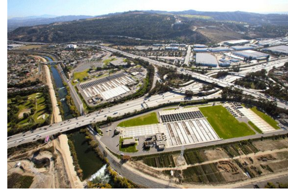
San Jose Creek WRP - 1972
