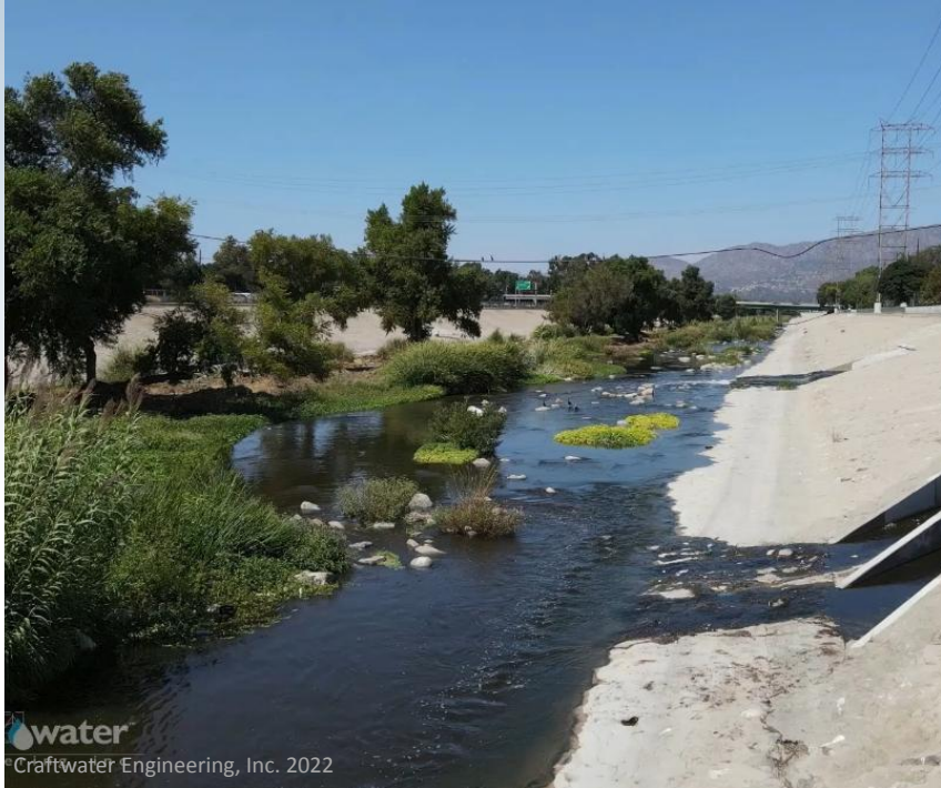
Storm Drain Discharge
