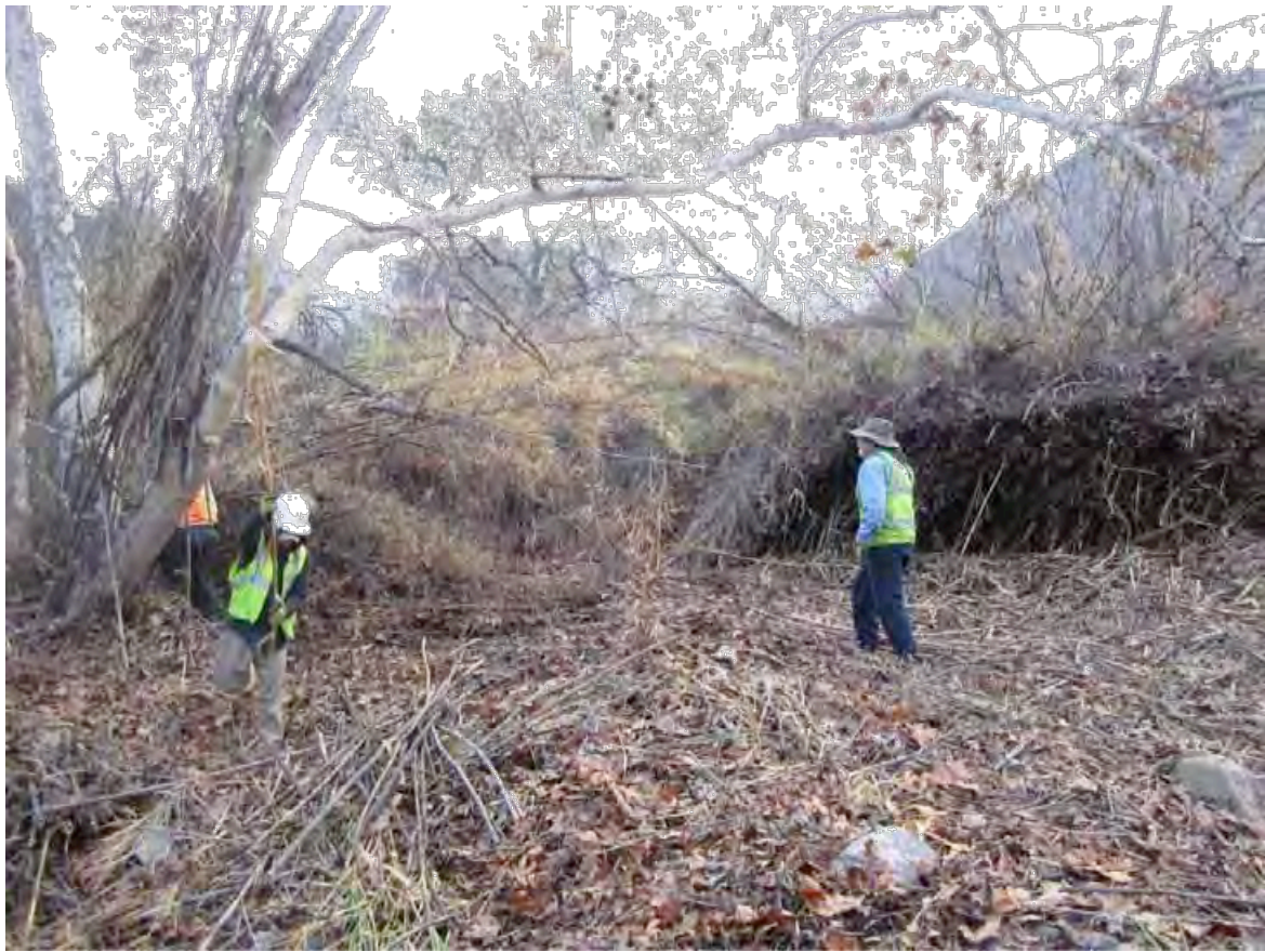
Photo point #2: Little Tujunga: 2016-11-1 Before cutting and chipping.
