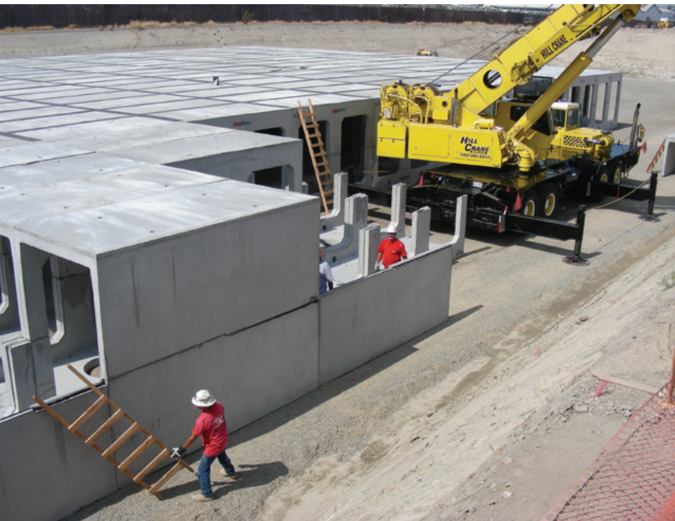
FIGURE 14 - DISCOVERY PARK INFILTRATION SYSTEM
